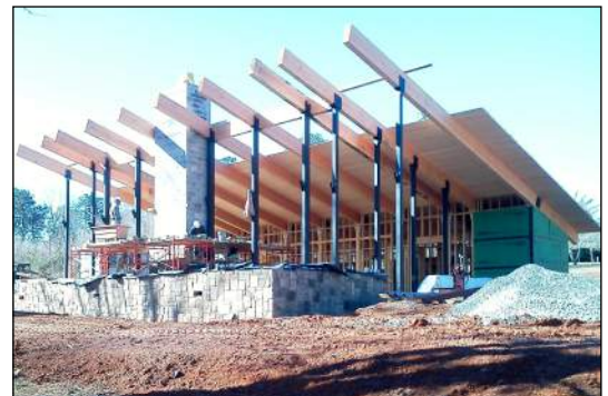
Auditorium taking shape - early February 2015. Photo by Kevin Hoyt.
