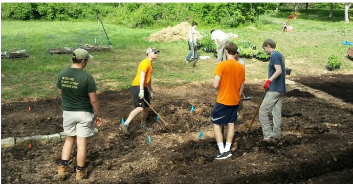
UT students working on the rain garden installation
