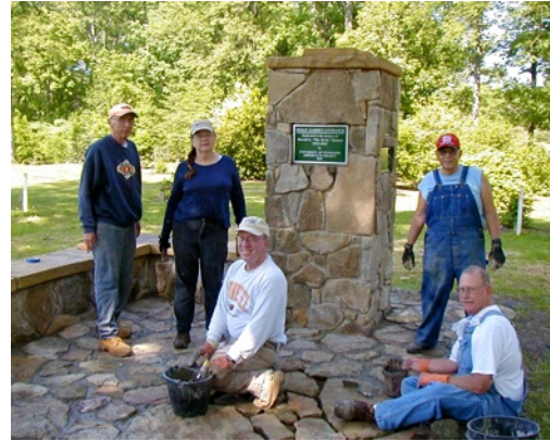
Applying mortar - one of the last steps - are Bob Reed, Lynn Carlson, Norm Dobbs, Carmen Gianforte and Chuck Haynes
